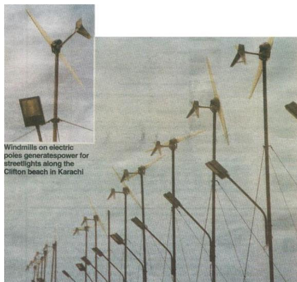
Figure 1: So-called wind farm installed at Karachi Beach and failed after few weeks.
